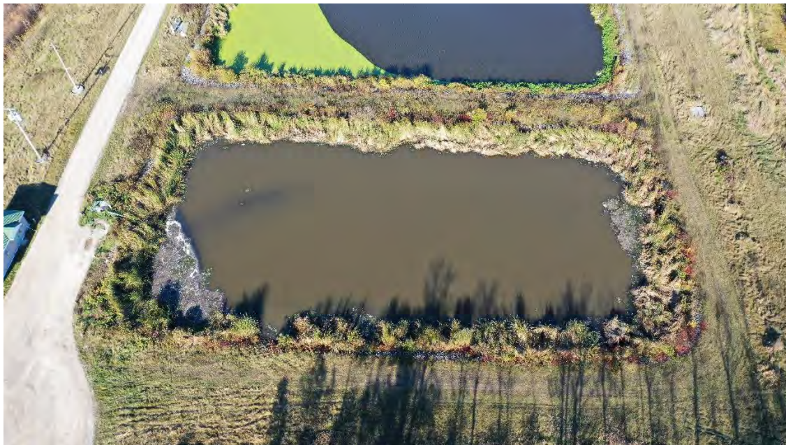
Aerial Drone Image. OCWA – Biosolids West Cell 1.
