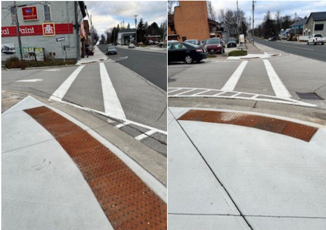
New curb ramps installed for the Lion's Head Sidewalk Project
