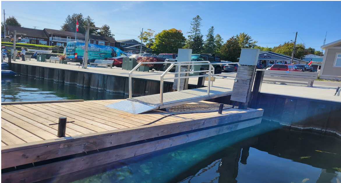
Ramp at the boat launch area at Little Tub Harbour
