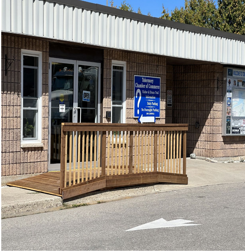
New access ramp in the Tobermory Chamber office
